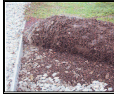
Figure II- 7. Drainage en gravillons (Source. Sopranature, Soprema, 2008)
