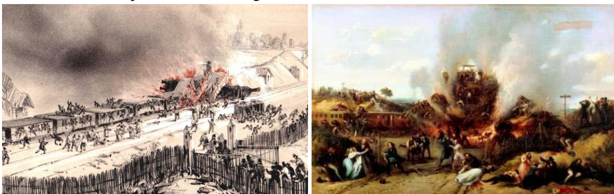
Figure I.9: Accident du train. [7]
