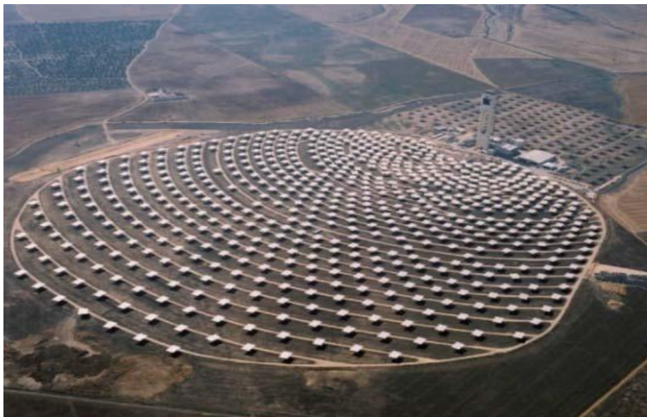
Figure II.9. Centrale tour solaire [2.17]
