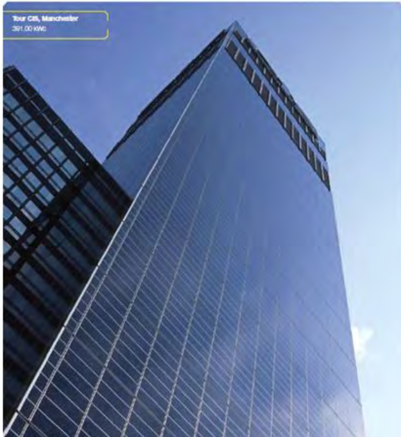
Figure 4.14 : La tour CIS. Manchester, UK, 391.00 kwc. Source : solarcentry
